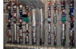
Prague Marina Office Center, Praha
