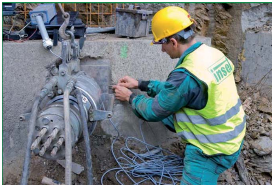
Obr. 15.1 - Monitoring kotev dynamometrem (foto: Inset)
